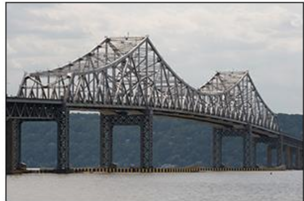
Tappan Zee Bridge
